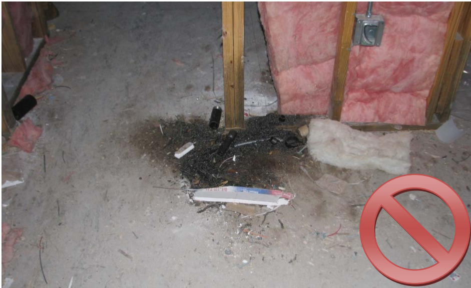
Photo of oil from a pipe cutter – this will create a problem with the floor underlayment and the final floor covering adhering properly.
