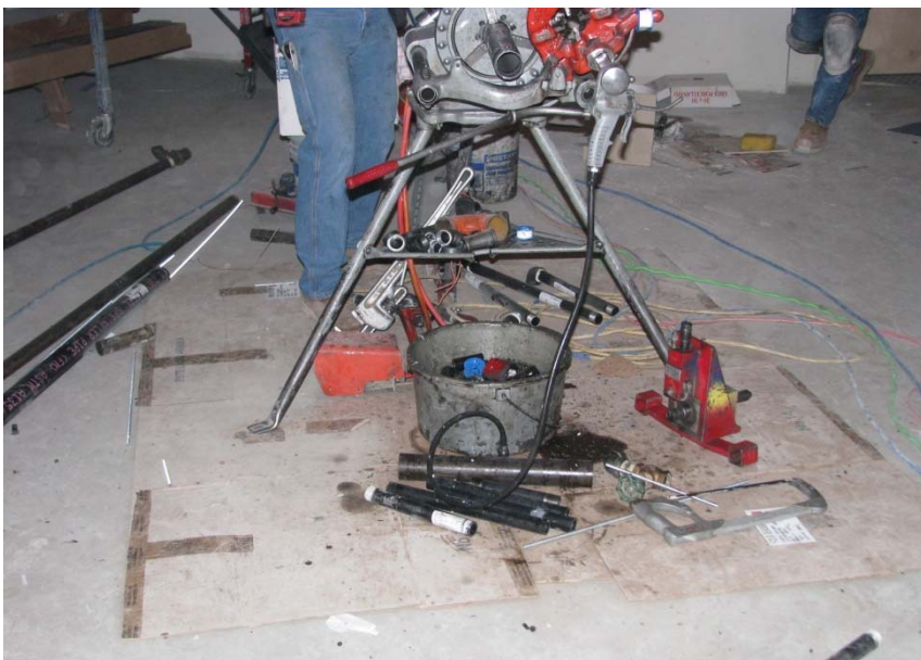
Photo of oil from a pipe cutter – this will create a problem with the floor underlayment and the final floor covering adhering properly.
